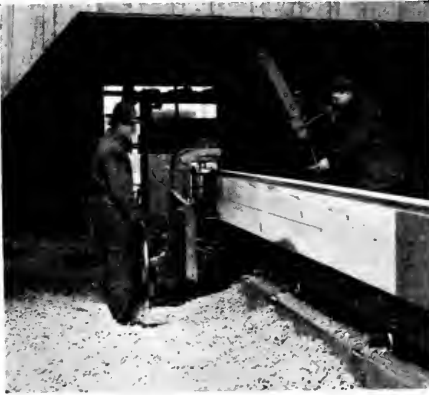
A patent planer at work dressing a keelson timber.
